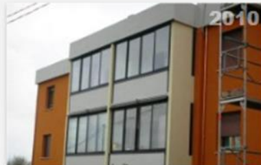
2010 Facade Restoration - Saltara - Residential
