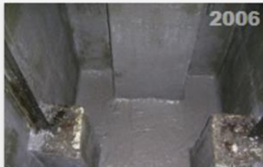
2006 Waterproofing of basements - Livorno - Residential
